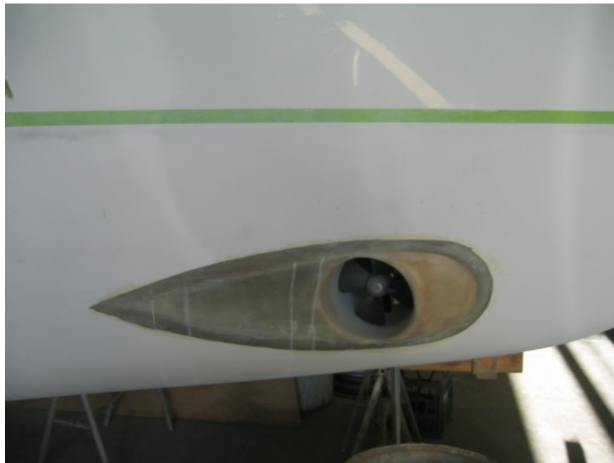
Fairing forward and aft of 6" bow thruster.
